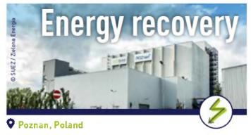
Under the form of a PPP and funded by EU Cohesion Funds, Poznan Waste-to-Energy plant will treat up to 210,000 tones of municipal waste originating from the 740,000 inhabitants of the region. The plant produces energy, partly renewable, in the form of electricity for the grid, and heat for the district heating network.
