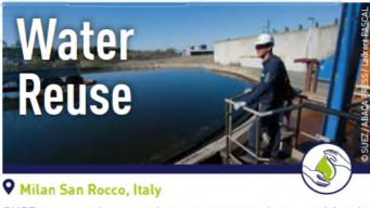
SUEZ set up a plant treating wastewater to be reused for the culture of rice in the Milan surroundings. In dry periods, all recycled wastewater is used to irrigate 22,000 hectares of crop fields.
