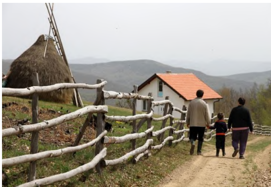
Family house built with the support of the RHP, allowing an internally displaced family to return to their native village in Bosnia and Herzegovina.
