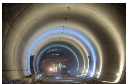
Tunnel T1 during construction
